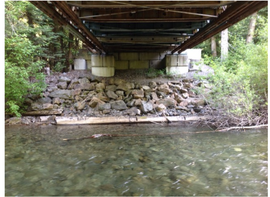
Right Bank Abutment when facing downstream
