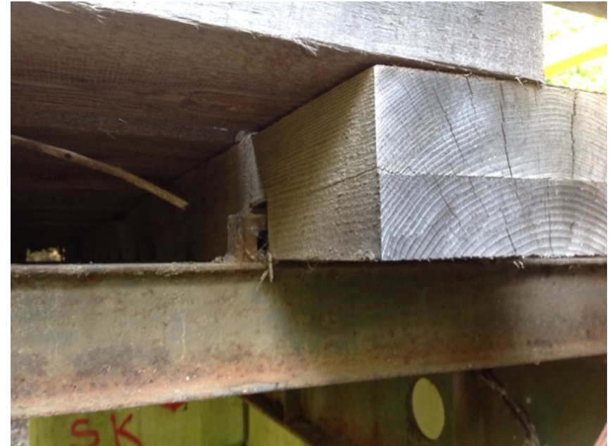
ties are notched to fit on stringers
