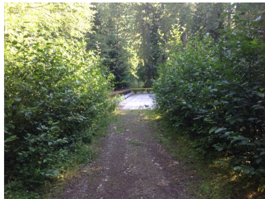
Approach from Left Bank when facing downstream
