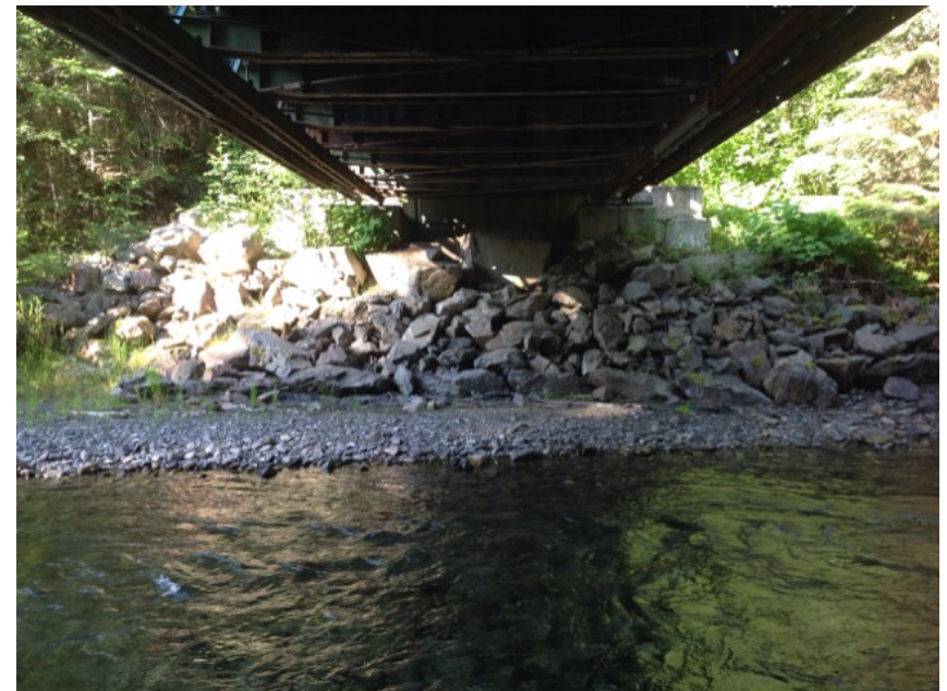
Left Bank Abutment when facing downstream
