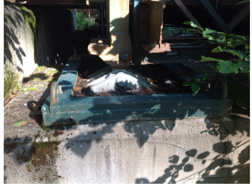
bearing plate - typical all 4 corners
