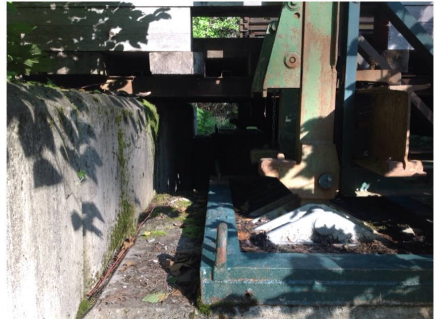
end post to ballast wall alignment
